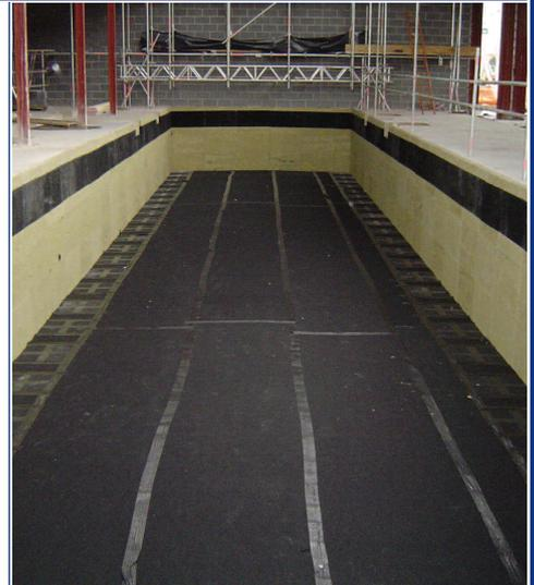
Regupol RAV materials were used to isolate the foundation of a KBA Commander Press
