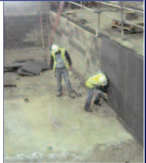
**CMS ISOSheet was used to achieve total sidewall isolation of two foundation pits.**
