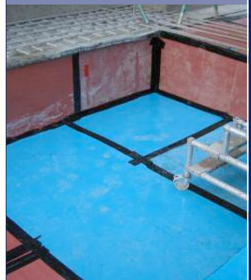
To ensure effective isolation, Regufoam materials were installed underneath the raft slab. With the development situated in a high water table, the level of which is just below the basement floor, any vibration control system specified had to be resistant to the effects of water penetration. As a dense closed cell foam, Regufoam was chosen because of its proven record of long term performance in similar water prone environments.
