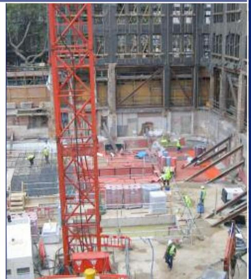
**CMS Vibrations isolated the foundations and basement walls at One Southampton Row using a combination of Regupol RAV and Regufoam materials.**
